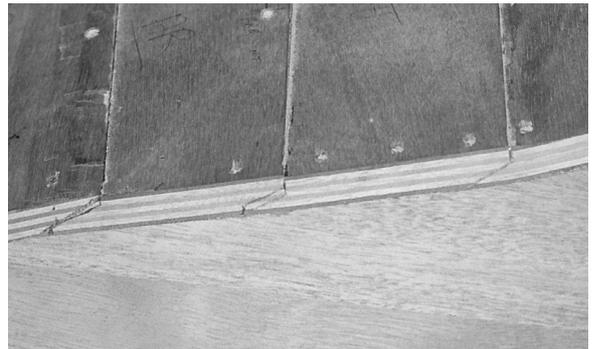
Whatever method is used, it is practical to fasten a temporary batten to guide the tools (picture).
