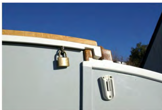
Padlocked descending panel
