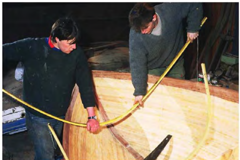
Installing a chord on an Aber - © Francis Holveck in Douarnenez
