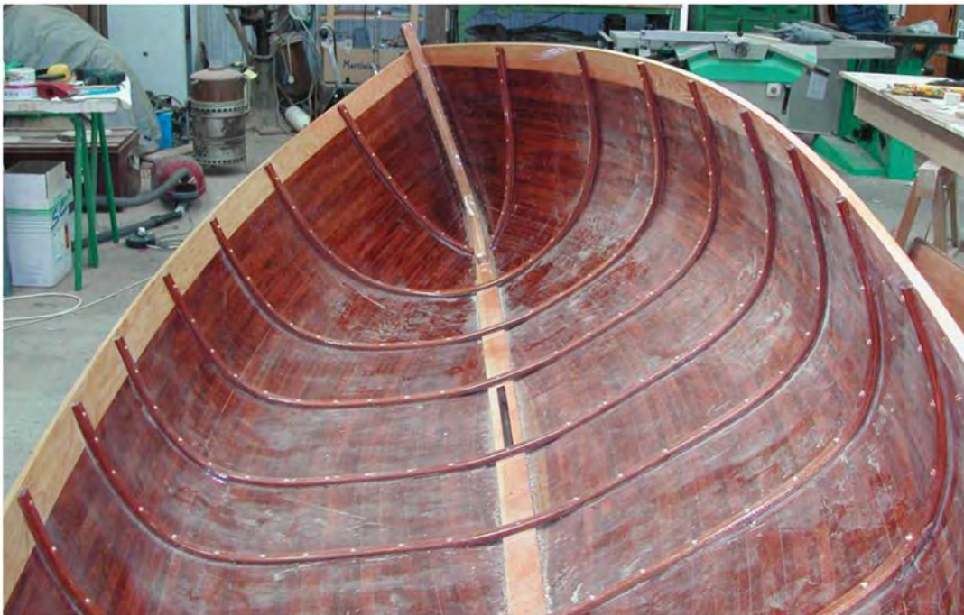
Hull after laying lamellated ribs in-situ © Jean-François Dockes
